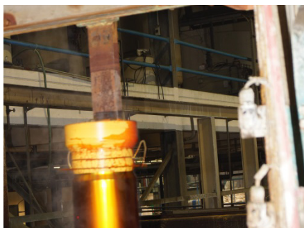
Photographs show (above) conventional return-type machines for mass production and (below) hoist lines at close range.
